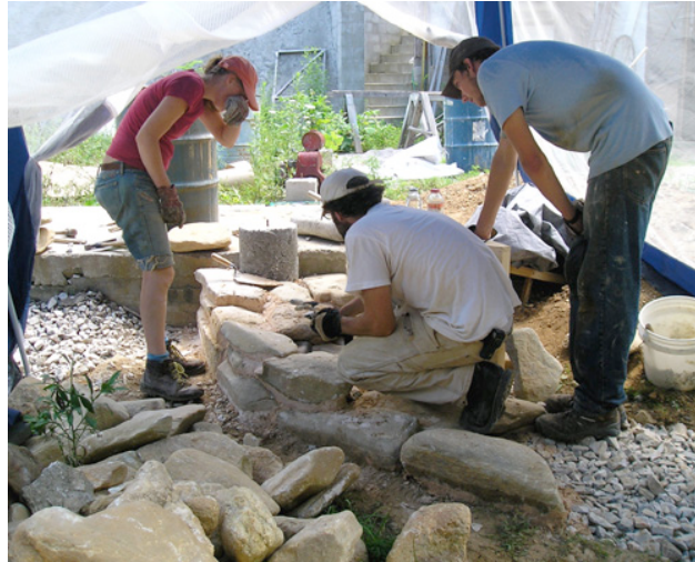
Dry-stacking stone for cob tower foundation
