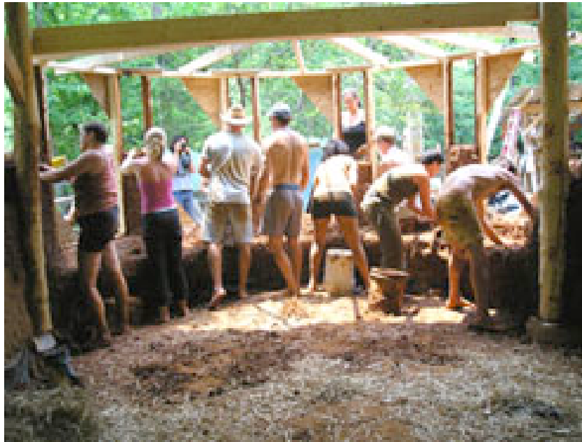
Interns in 2007 build a cob wall at Leela House.
